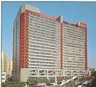
Tuen Mun Plant (Hong Kong)
